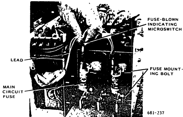
Fig. 17 Main Circuit Fuse (230V, 25A)
