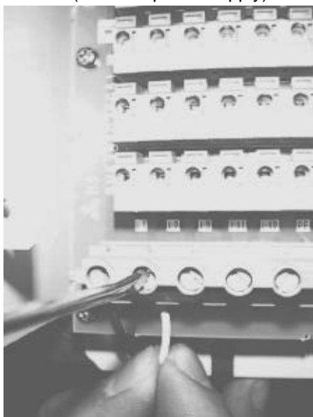
Insert the wire, and tighten the terminal with a flat-tip screwdriver. The tightening torque is 0.5 to 0.6Nm.
